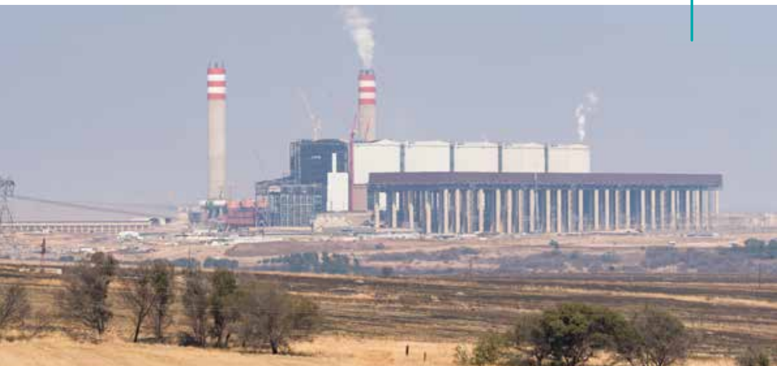
Eksom's Kusile power station, Mpumalanga. (Photo: Childa Santrucek / Alamy Stock Photo)
